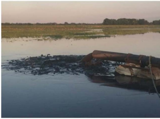
Figure 25. Dredged reservoir sediment being used for soil augmentation at John Redmond Reservoir, KS.
