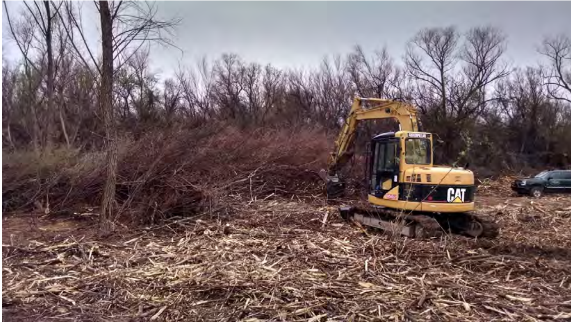
Figure 2 - Excavator with mulching head chipping Tamarisk slash piles
