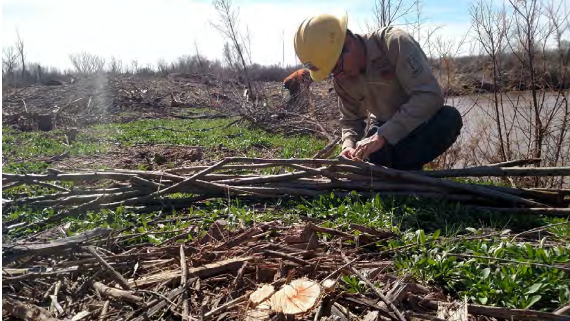
Figure 3 - Arizona Conservation Corps crewmembers installing willow bundles in Ft. Thomas
