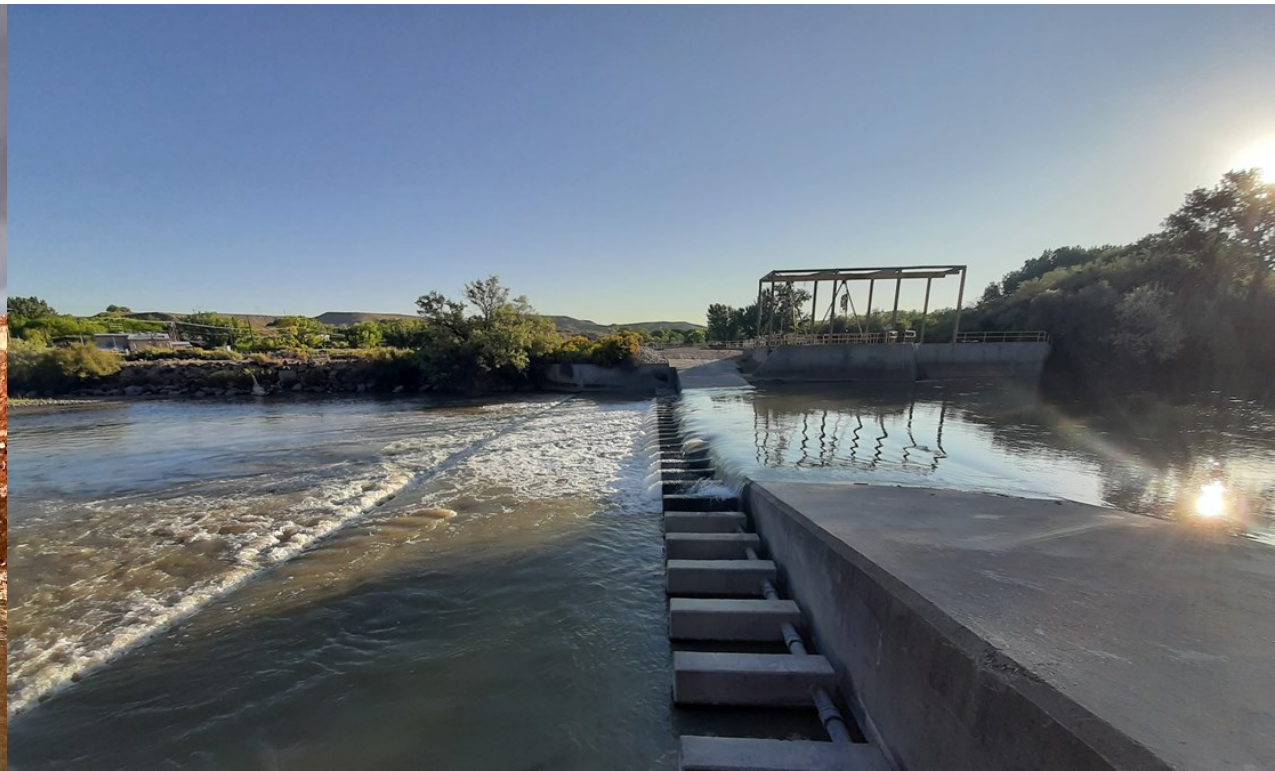
Public Service Company of New Mexico (PNM) weir
