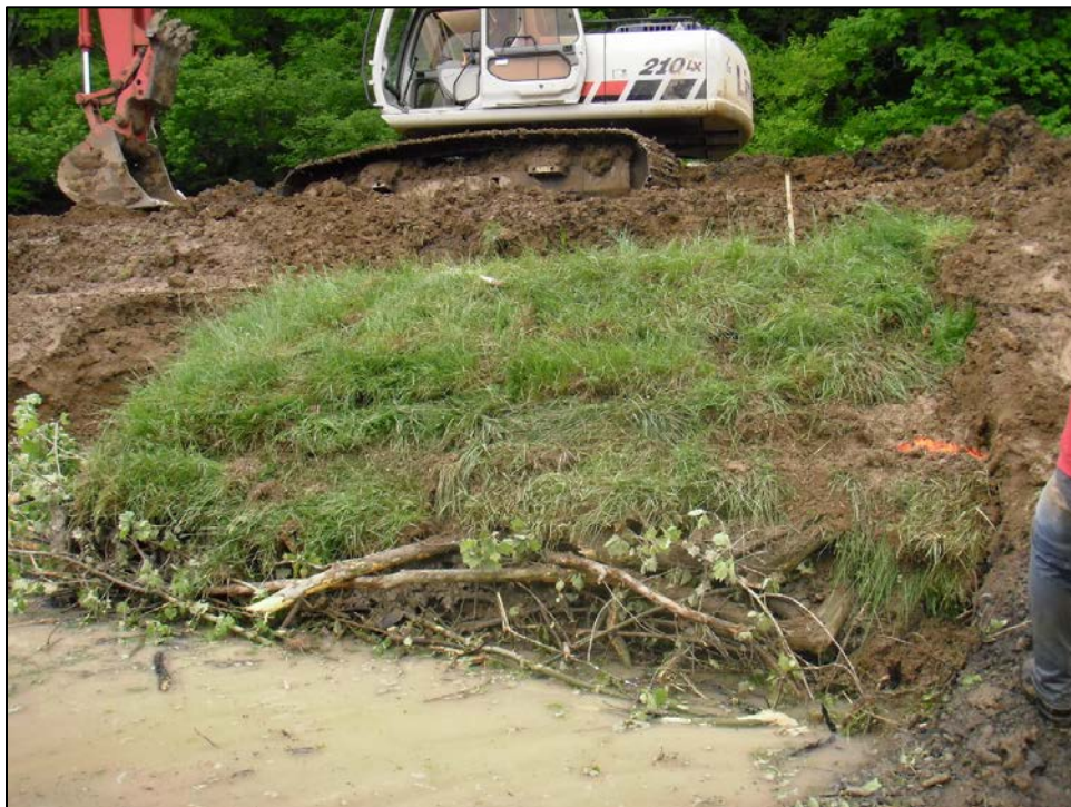
Figure 10. Woody debris and toe sod mat combo BMP. Photograph courtesy of Stantec Engineering.
