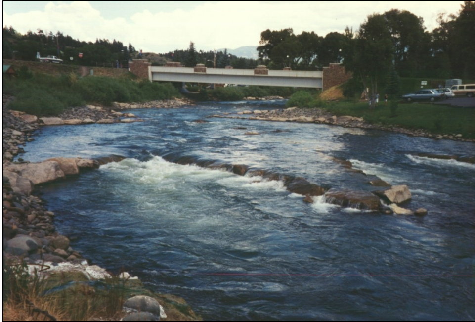
Figure 7. W-weir BMP. Photograph courtesy of Wildland Hydrology.
