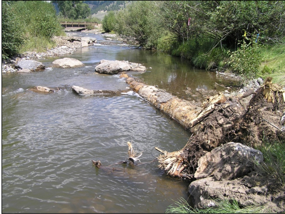
Figure 9. Rootwad and log vane combo BMP. Photograph courtesy of Stantec Engineering.
