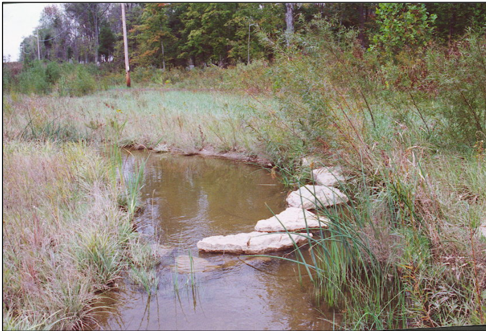
Figure 8. J-hook BMP. Photograph courtesy of Wildland Hydrology.
