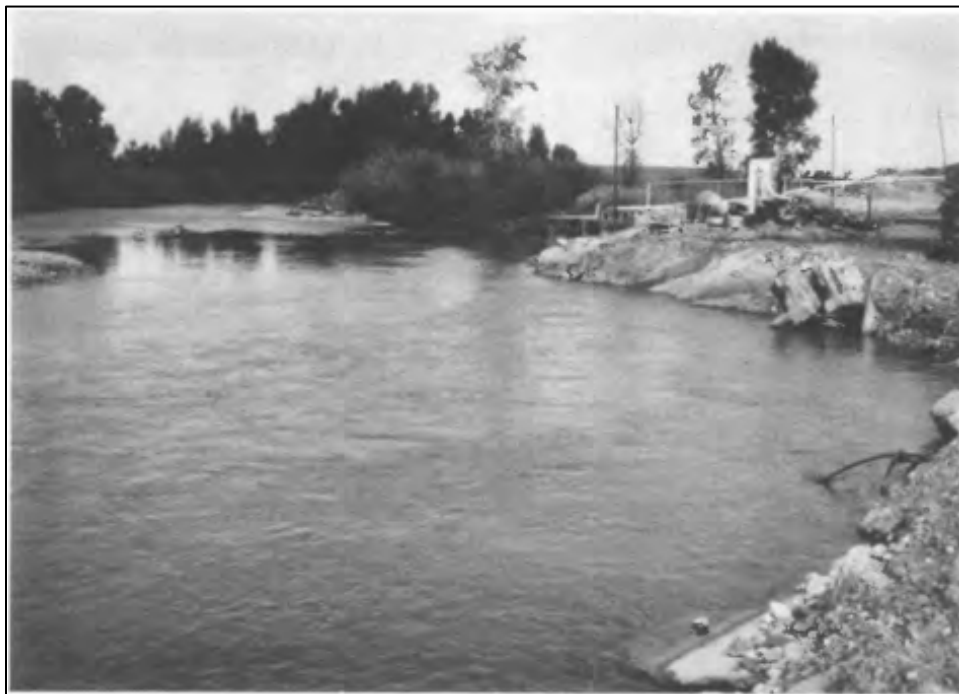
Figure 2. Riprap bank stabilization on the Bear River near Evanston in 1983. Photograph courtesy of Smith and Maderak (1993).
