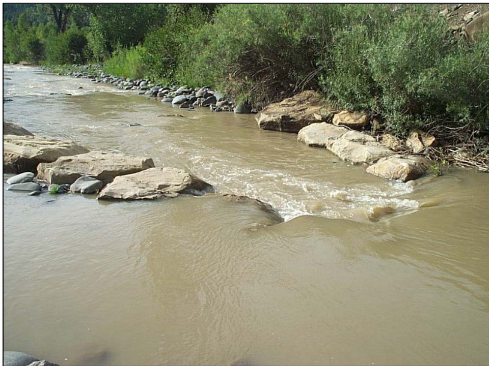
Figure 6. Cross-vane BMP. Photograph courtesy of Wildland Hydrology.
