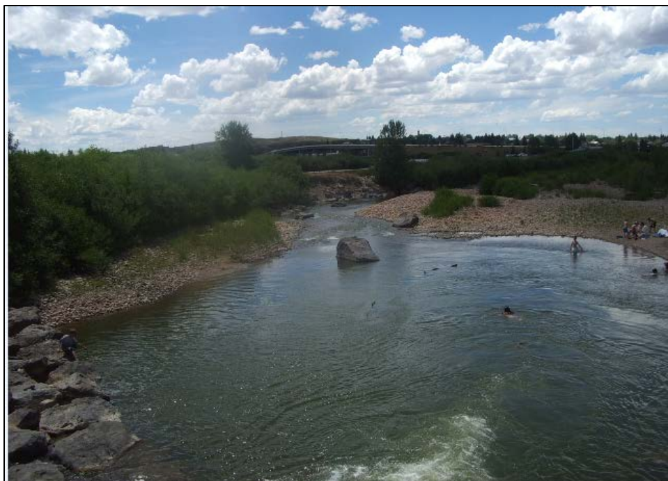
Figure 5. Boulder placement and channel stabilization - City of Evanston Greenway.
